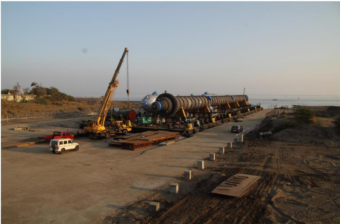
CCR is the key process in oil refinery converting low value naphtha to high valuable products like Petrochemicals and Gasoline through various reactions such as Dehydrogenation, Aromatisation, Isomerisation, Dealkylation, Dehydrocyclization. The CCR Reactor is a tall column like equipment with continuous moving catalyst. Very stringent tolerances are required
